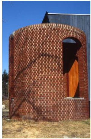
Brick entrance drum above a 6' cistern with roof-collected water.
